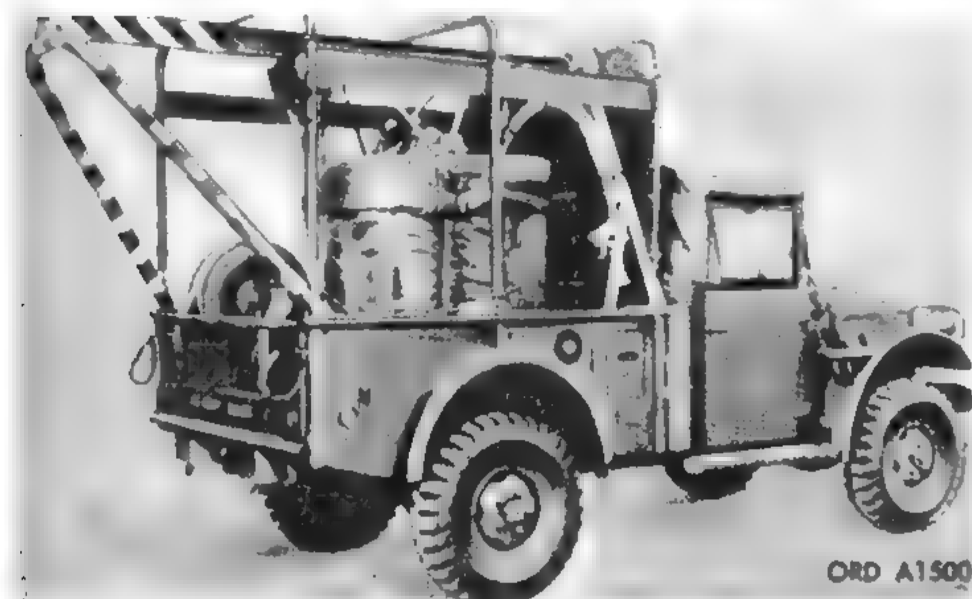
Although the M506 resembles a WWII era bomb truck, in fact it was a hydrogen peroxide servicer for the Redstone missile system.
